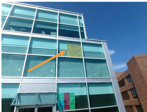
Photo 3.1-16: Broken IGU panels are present. Damaged glass is not prevalent; however, it is present in at least two locations.
