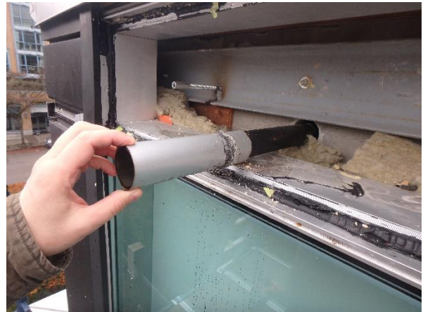
Photo 3.3-4: The water ingress path between the scupper pipe (black) and the decorative sleeve (silver).
