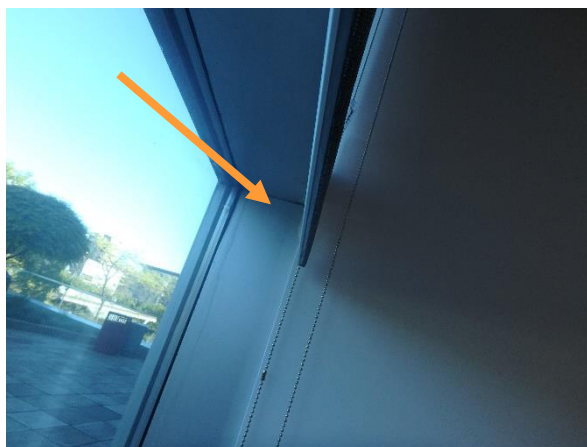
Photo 3.1-23: Drip marks on the curtain wall's horizontal elements – 3 rd floor office.
