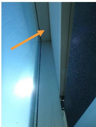
Photo 3.1-22: Signs of water run-offs at the 3 rd floor curtain wall interior frames.
