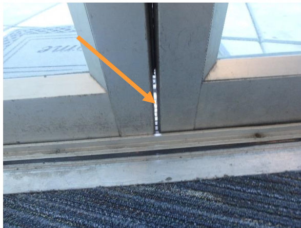
Photo 3.1-28: Damaged and difunctional weather-strips at the southernmost 3 rd floor tierce door.
