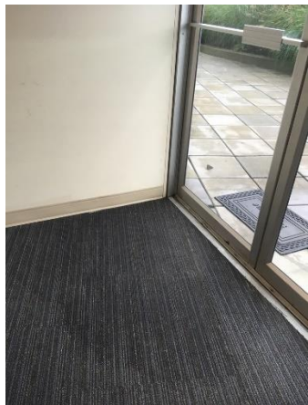
Photo 3.1-27: Wet carpet due to water ingress through the southernmost 3 rd floor terrace door.
