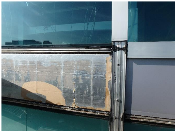
Photo 3.1-20: Aged and partially degraded insulation panel at the 3 rd floor mock-up repair.
