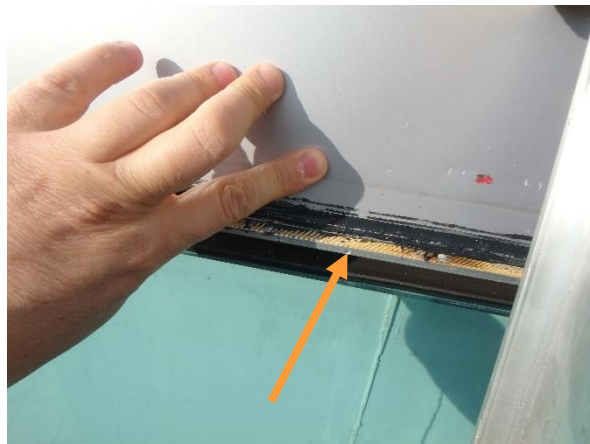
Photo 3.1-14: Water accumulation behind the spandrel was observed. A significant amount of water flowed out once the sheet metal covers were removed.
