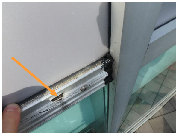
Photo 3.1-12: Plugged pressure plate weep holes were observed at the repair mock-up area.
