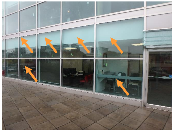
Photo 3.1-18: Area with the majority of the failed IGUs at the 3 rd floor terrace.
