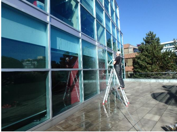
Photo 3.3-1: Water testing of the repair mock-up at the 3 rd floor.
