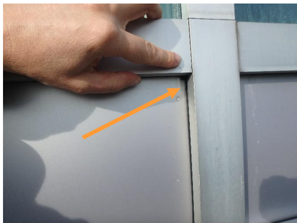
Photo 3.1-11: A significant amount of water accumulated under the beauty caps. The cap weep holes were observed to be plugged.
