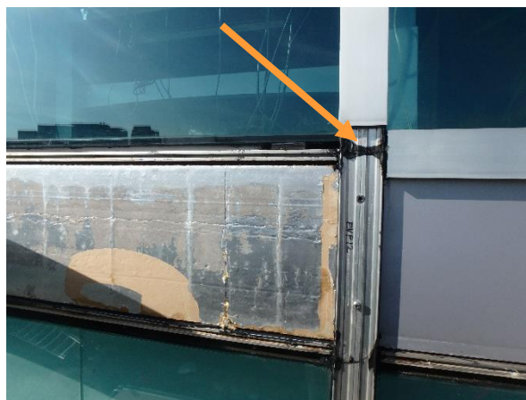
Photo 3.1-8: Sealant at the vertical pressure plate ends was observed to be split.
