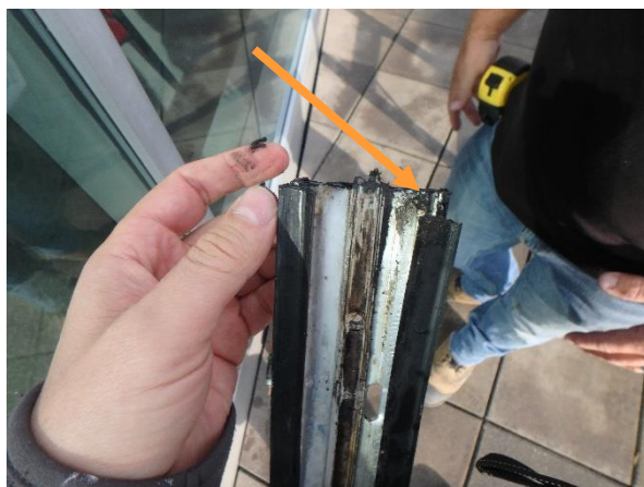
Photo 3.1-5: Short gasket at pressure plate end.
