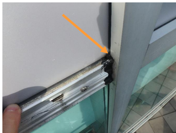
Photo 3.1-4: Gap at the pressure plate end due to shrunken gasket. The gaps at the gasket ends allow water into the glazing cavity.
