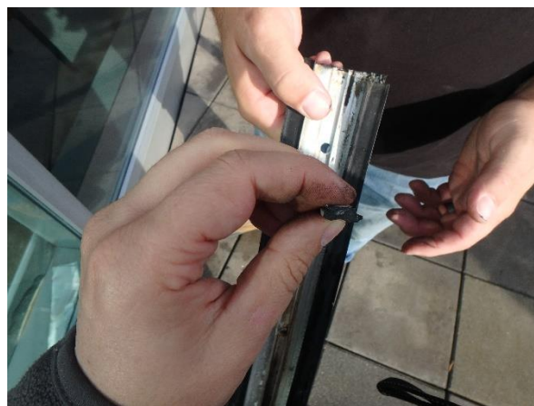
Photo 3.1-6: The middle gasket at the pressure plate appeared to prevent proper plate compression.
