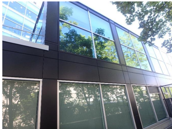
Photo 2.1-2: General view of the storefront windows at the ground floor. Note: A curtain wall system forms the enclosure at the 2 nd floor in this photo.
