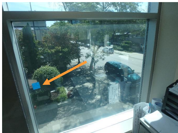
Photo 3.1-15: Failed IGUs were marked by the owners with stickers.
