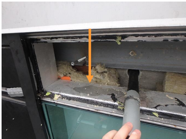
Photo 3.1-26: Water accumulation at the curtain wall horizontal rail at the 2 nd floor kitchen assembly.
