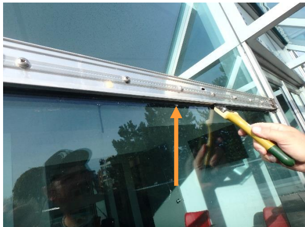
Photo 3.1-13: Water accumulation under pressure plates was observed. A significant amount of water flowed out after the plates were removed.
