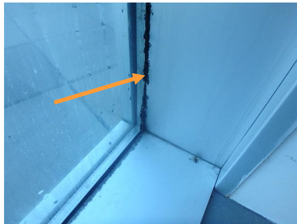
Photo 3.1-10: The interior sealant bead at the glass / frame perimeter shows signs of flowing and displacement.
