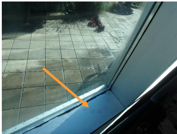
Photo 3.1-23: Drip marks on the curtain wall's horizontal elements – 3 rd floor office.
