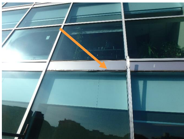
Photo 3.1-7: Sealant at the spandrel panel sheet was observed to be discontinuous.
