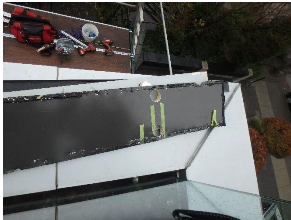
Photo 3.1-21: Spandrel panel in relatively good condition removed at the 2 nd floor kitchen ceiling localized repair.
