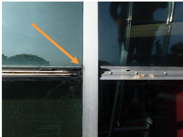
Photo 3.1-9: Sealant at the frame horizontal connection was aged and dysfunctional.
