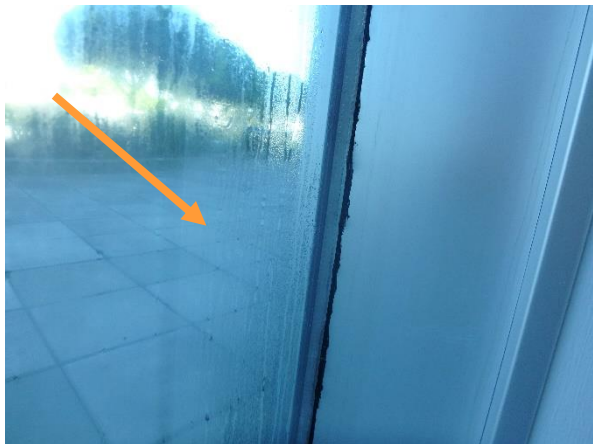
Photo 3.1-17: Condensation forming between the glass panes denoting failed IGU.
